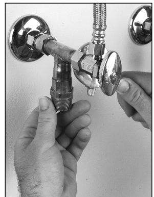
2. Install tees and attach angle stops.
